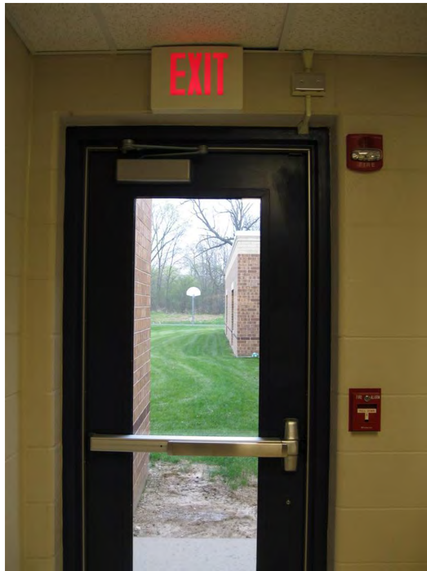
Typical Exterior Door
