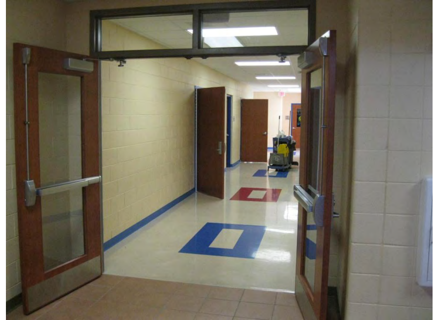
View of Common Corridor
