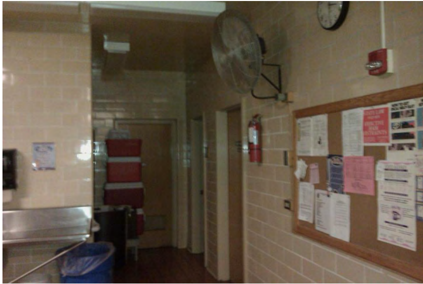
View of Kitchen
