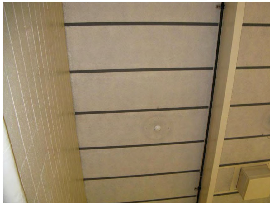
Gymnasium Ceiling with Typical Tectum Ceiling Panels
