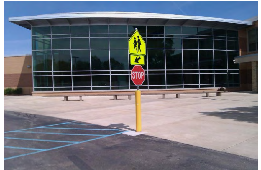
Performing Arts Center Glass Curtain Wall
