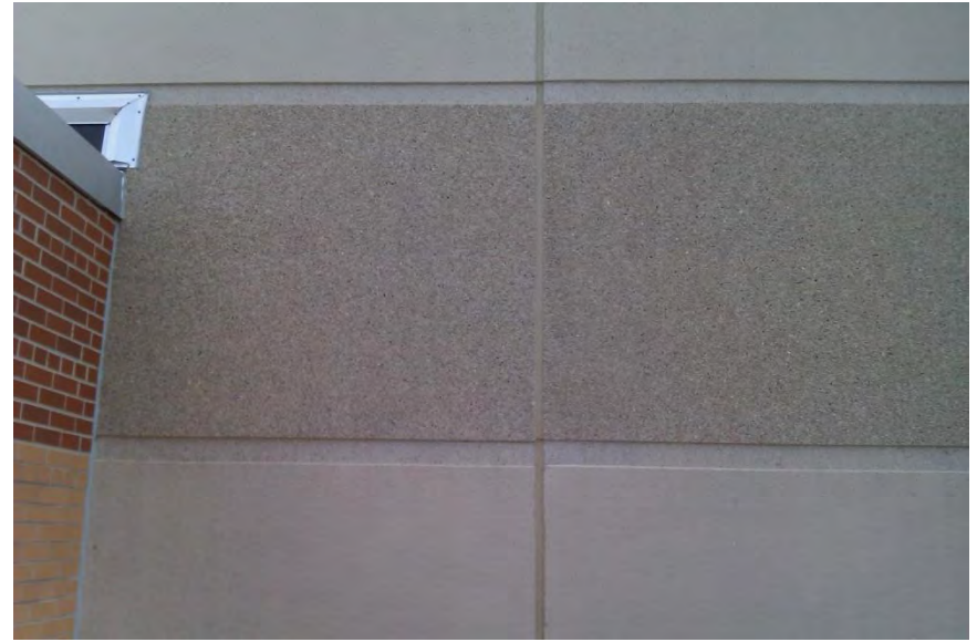
View of Precast Wall Panels
