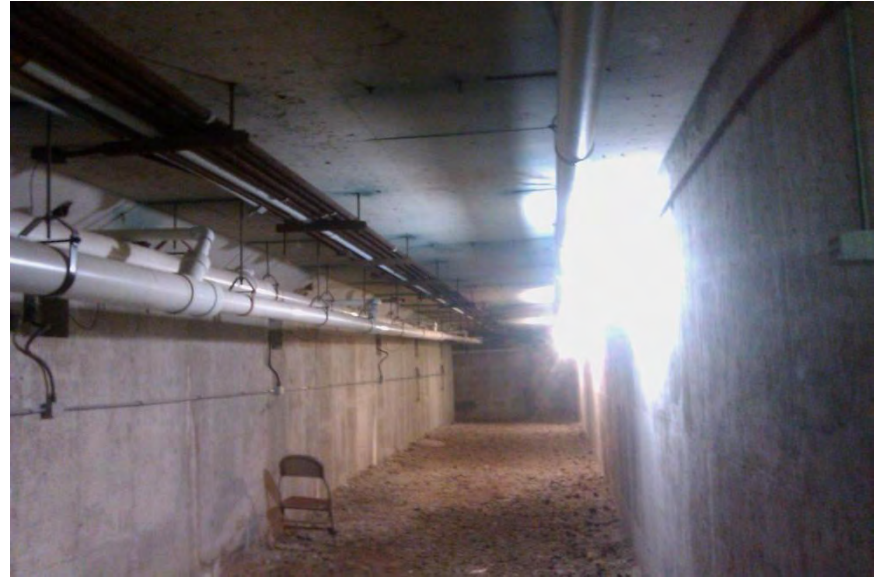
Swimming Pool Below Ground Corridor
