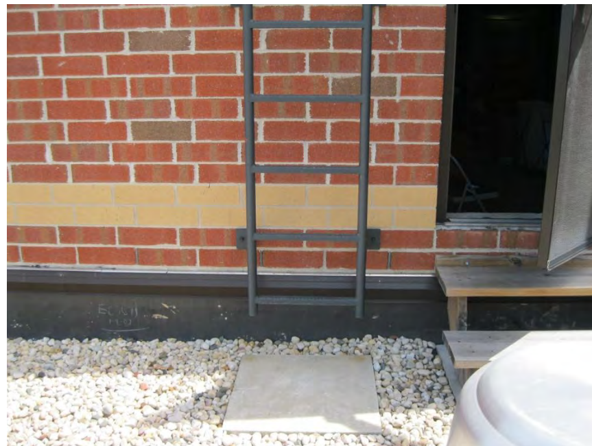
Mechanical Room Roof Access
