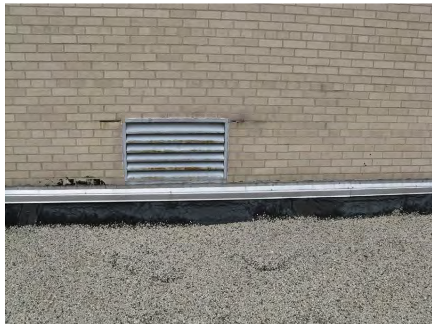
Ballasted Roof Showing Membrane Termination Detail and Vent
