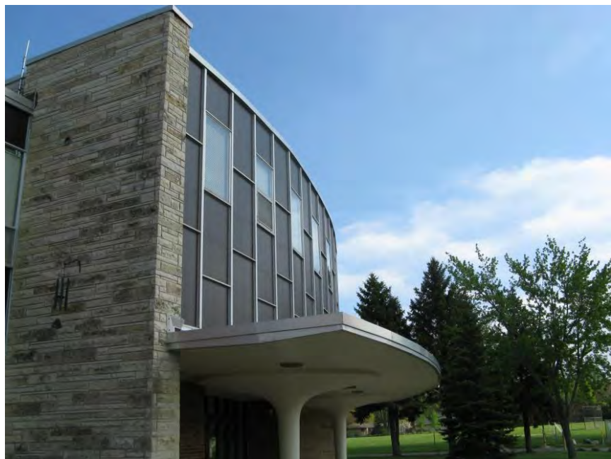
View of Front Facade
