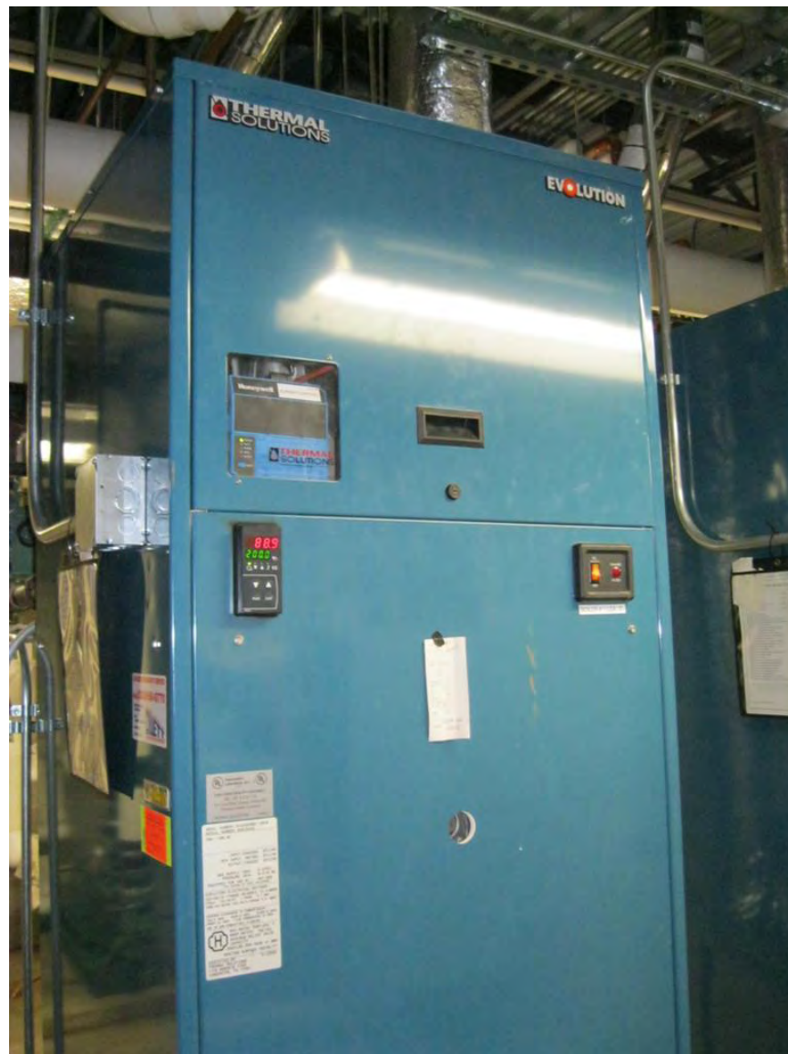
Thermal Solutions Boiler
