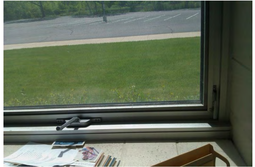
Typical Older Window
