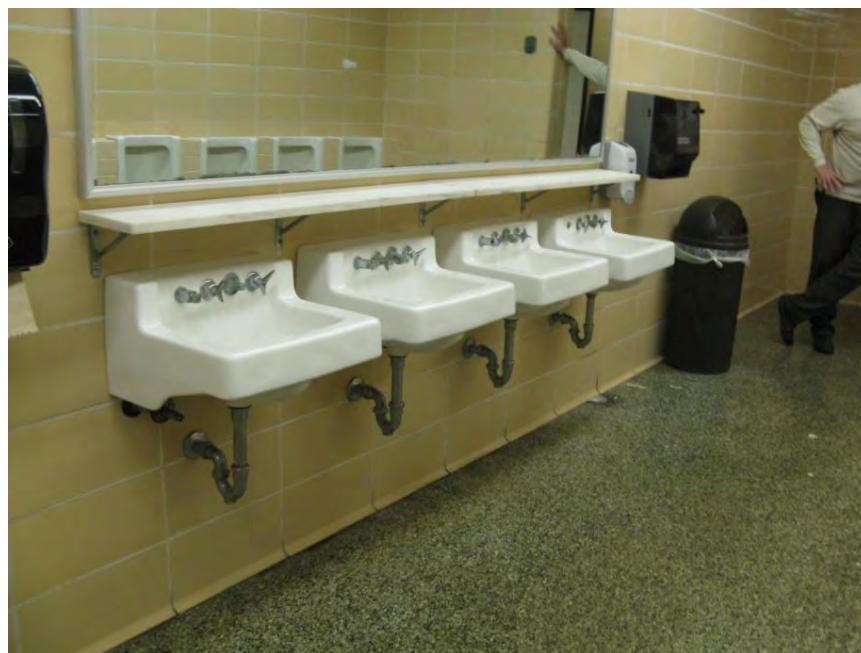
Typical View of Bathroom
