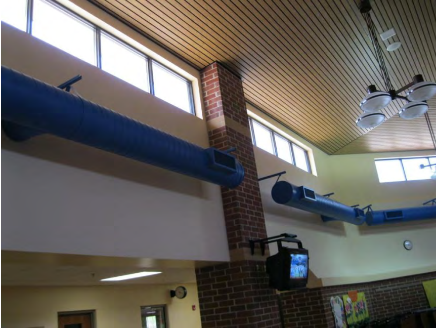
Commons Area Clerestory Windows, HVAC Ducts & Ceiling
