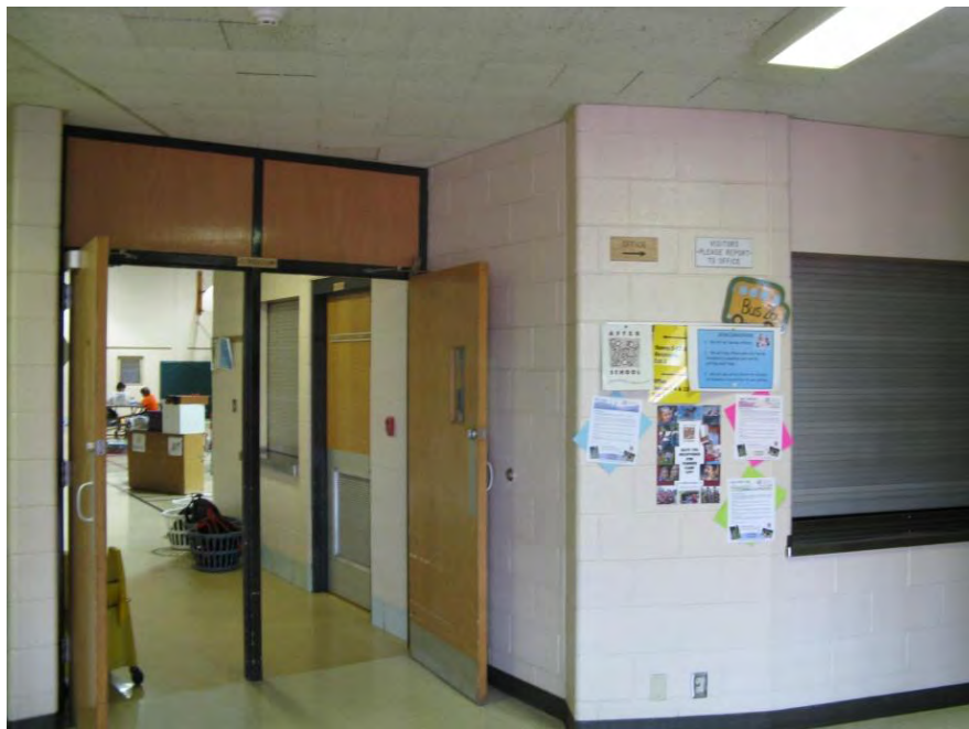
Typical View of Gymnasium Doors
