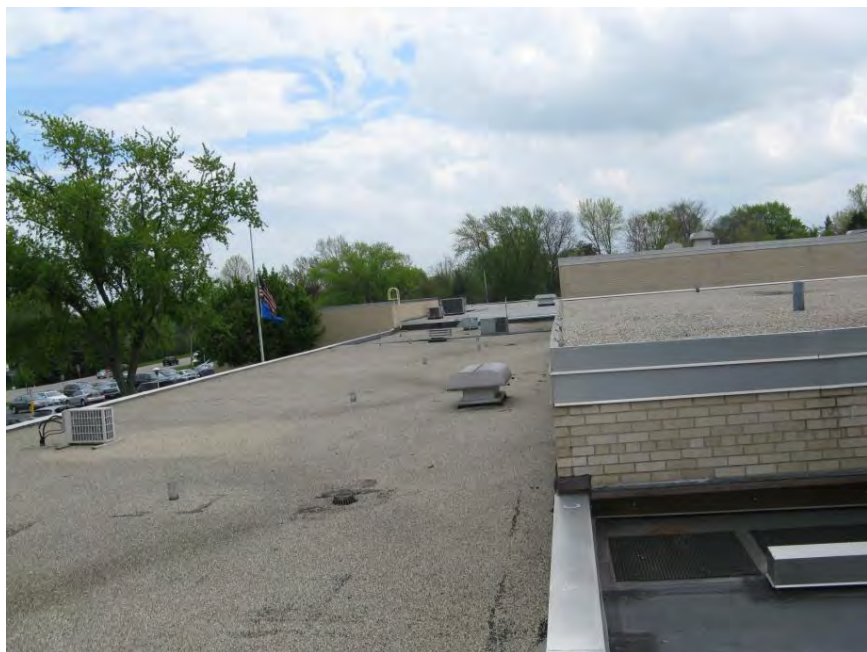
Ballasted Roof (left) and Adhered Roof (right bottom)
