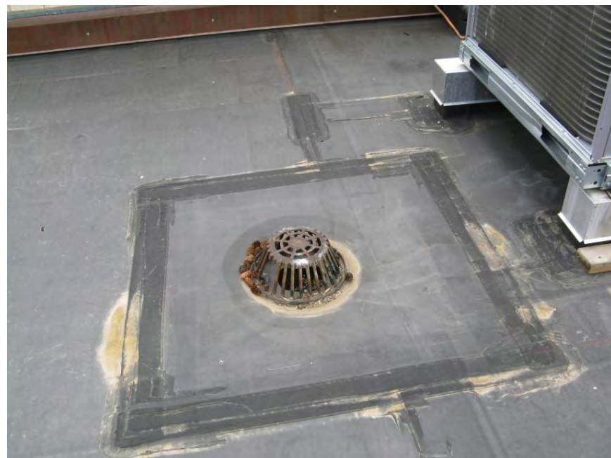
Typical Roof Drain
