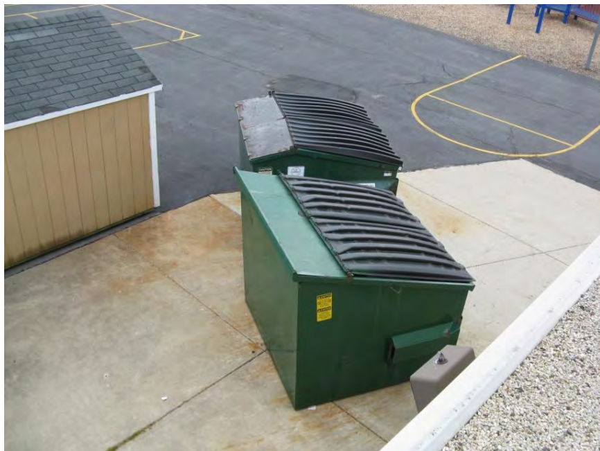
Trash Containers Lacking Enclosure
