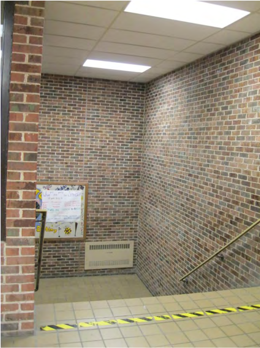
View of Stairwell
