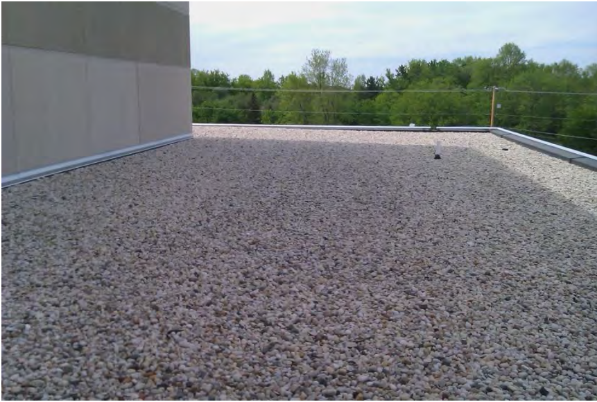
Ballasted EPDM Roof
